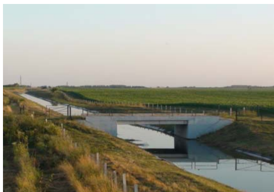
Figure 3: The second bridge (B2) at the 2+500 km
