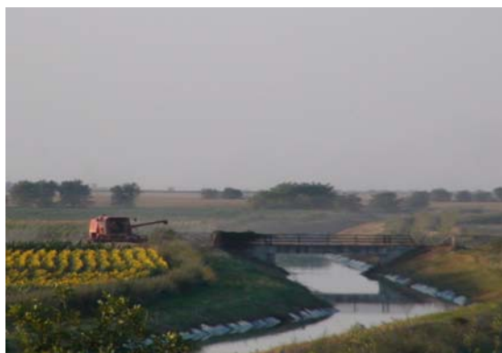
Figure 4: The third bridge (B3) at the 3+350 km
