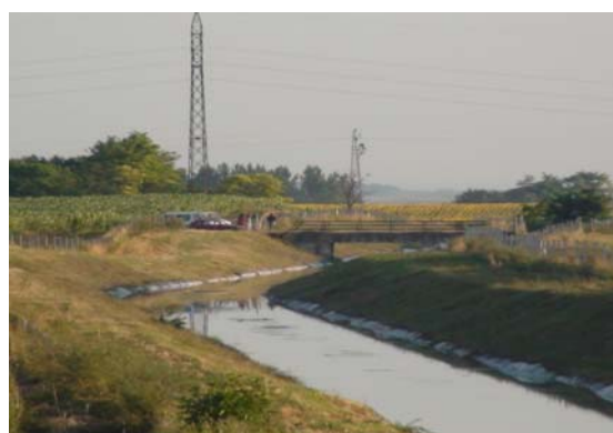
Figure 2: The first bridge (B1) at the 1+700 km
