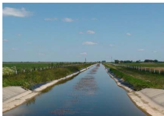
Figure 1: Lined irrigation canal “Kula-Mali Idoš” (start)
