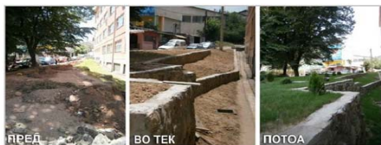
Figure 1: Construction of a new fountain and the Park of Generations in high school Vančo Prke in Štip (before, during and after the greening)
