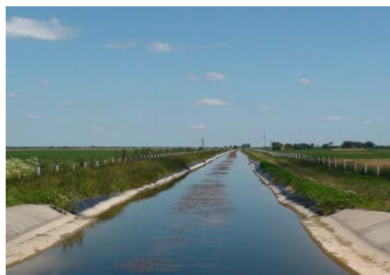
Figure 1: Lined irrigation canal “Kula-Mali Idoš” (start)
